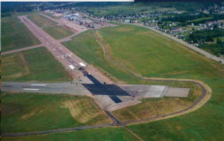
Paving the runway intersection
